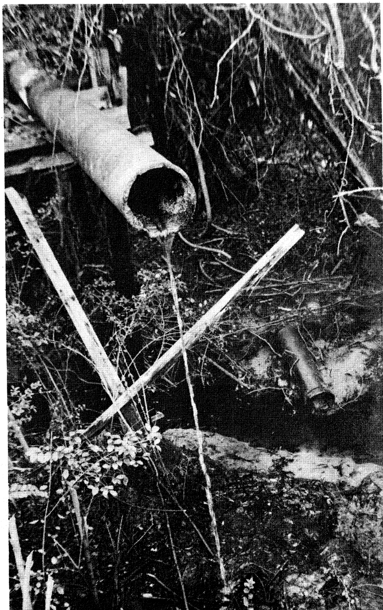
photo by Clint Schemmer Storm drain carrying rainwater mixed with raw sewage empties into King's Creek, Holly Ridge, Onslow County.
